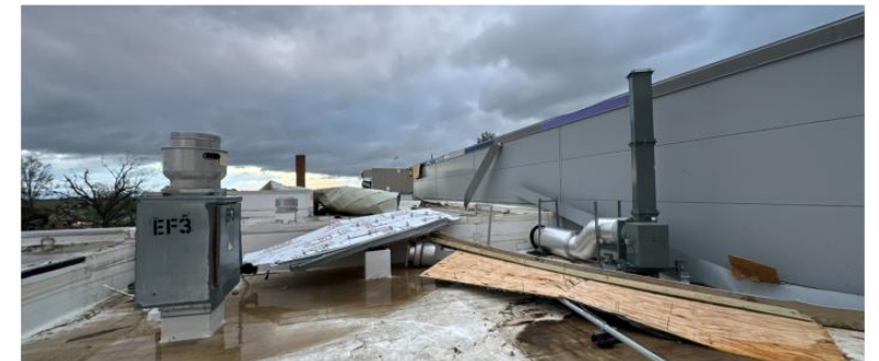
Roof / building envelope
